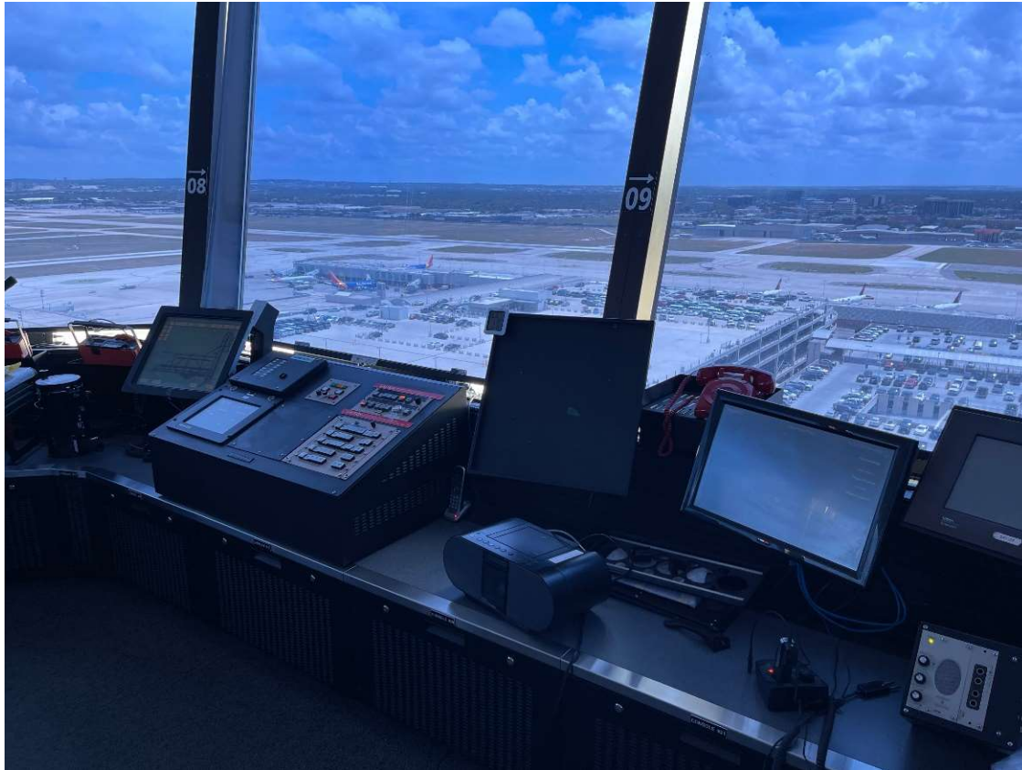
RIPSA Kill Switch will be between positions 7 & 8
